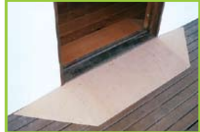
Timber wedge built by tradesperson
