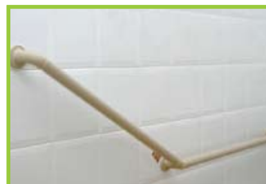
Grab rails on wall
