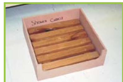
False draining floor
